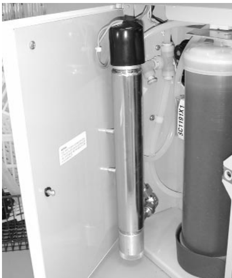
UV Lamp Installation
